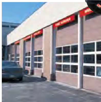
▲ As customers expand their service menu, Myers adapts to supply products they need to stay competitive— such as above-ground lifts that install without excavation to create new service bay space.
